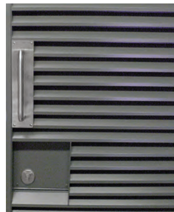
Typical lock and handle arrangement
